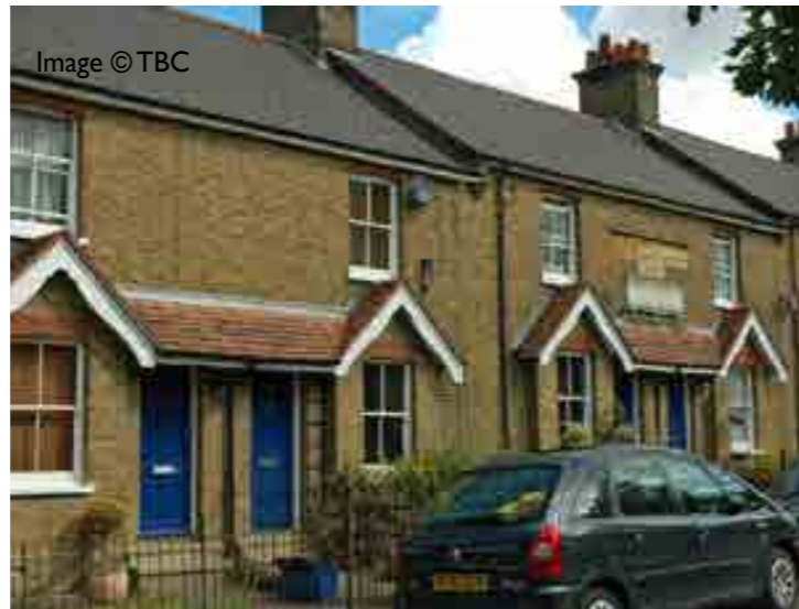
Articulated windows on Oddfellows Terrace, Old Harlow
