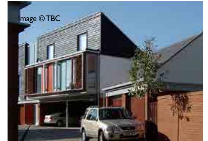
Image © TBC Innovative housing, Abode Newhall, Harlow
