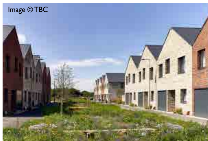
Strong terraced rhythm through repeated roof forms at St Chads, Tilbury, by Bell Phillips Architects
